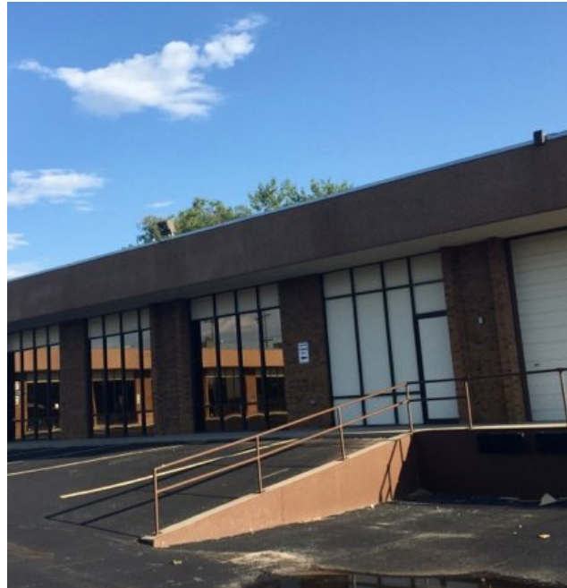
OVERHEAD DOOR BAY
