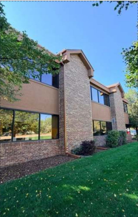
EAST ELEVATION & GROUNDS
